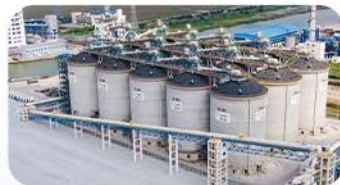
Silo Storage and Conveying
